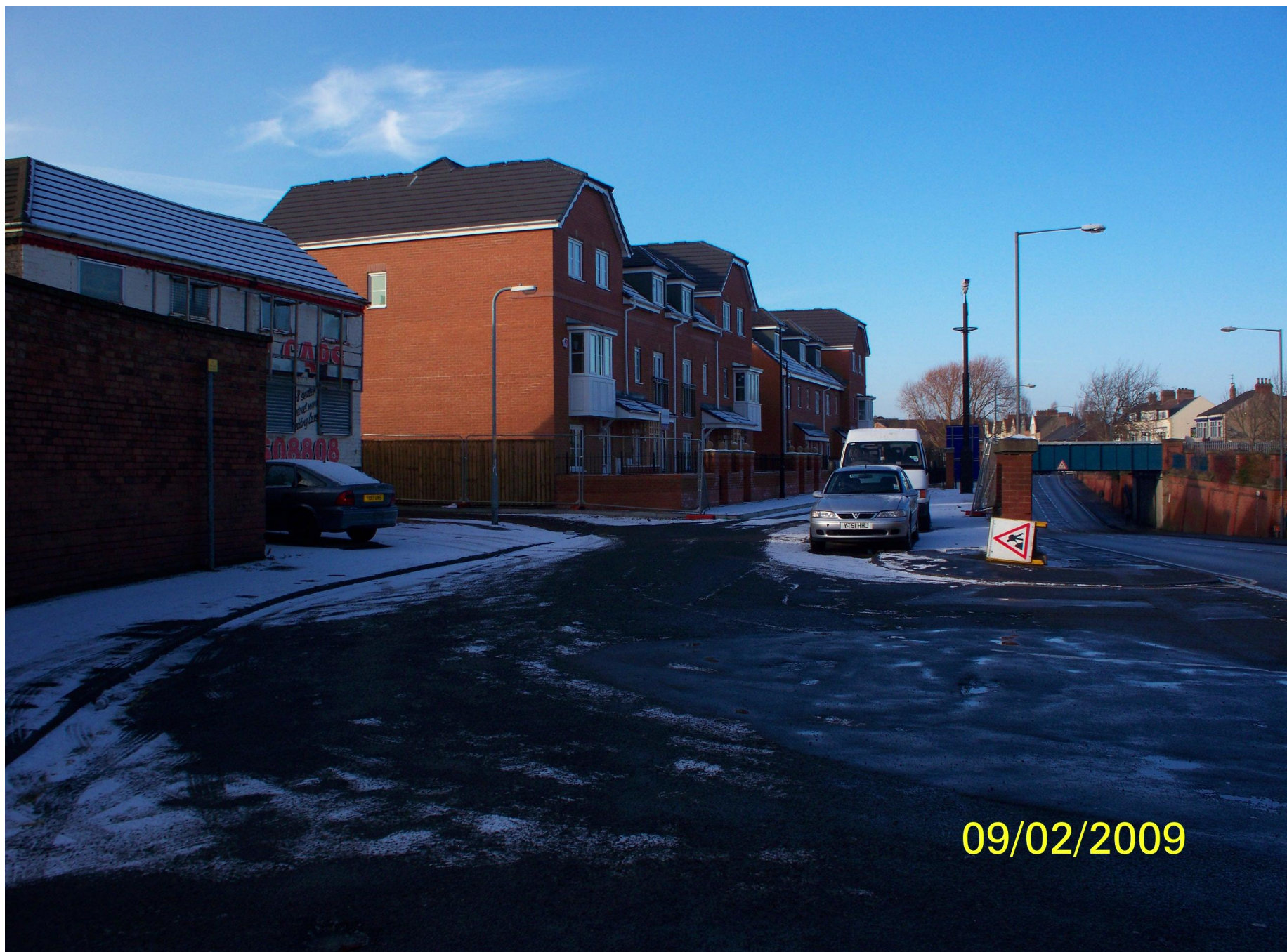
Vyner Terrace, Tees Valley cars premises, access to rear lane and approach to collapsible bollards.
